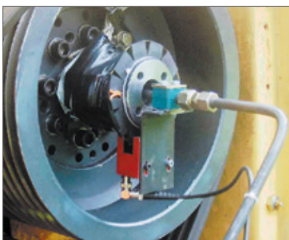
Measurement of vibration and torque through telemetry at side
