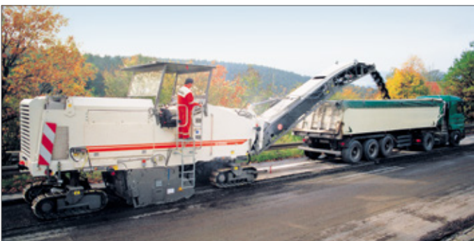
Road Milling Machine
